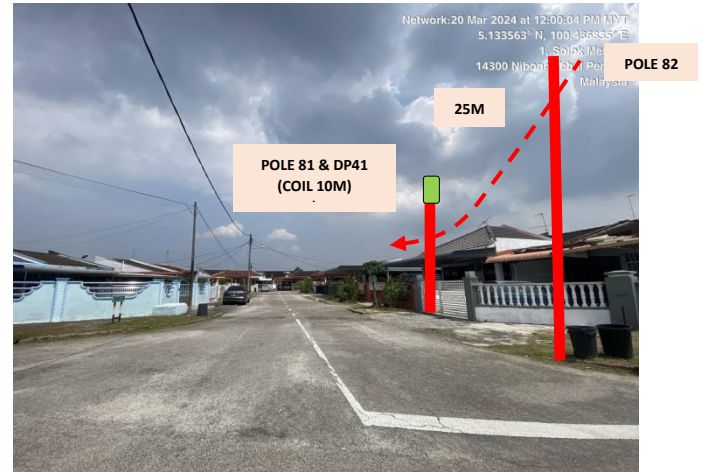
Picture 6 – JALAN SOLAK MERPATI BETWEEN UNIT 1 & 2
