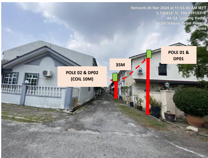
Picture 7– JALAN LINTANG KEDIDI 2 BETWEEN UNIT 54 & 53
