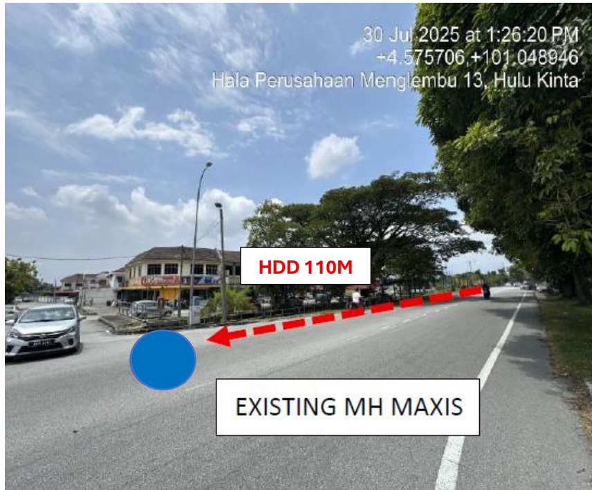
PICTURE 5 : HDD 110M TO EXISTING MAXIS MH
