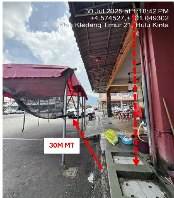
PICTURE 1 : TRENCHING 30M TO PROPOSE NEW MAXIS MH01
