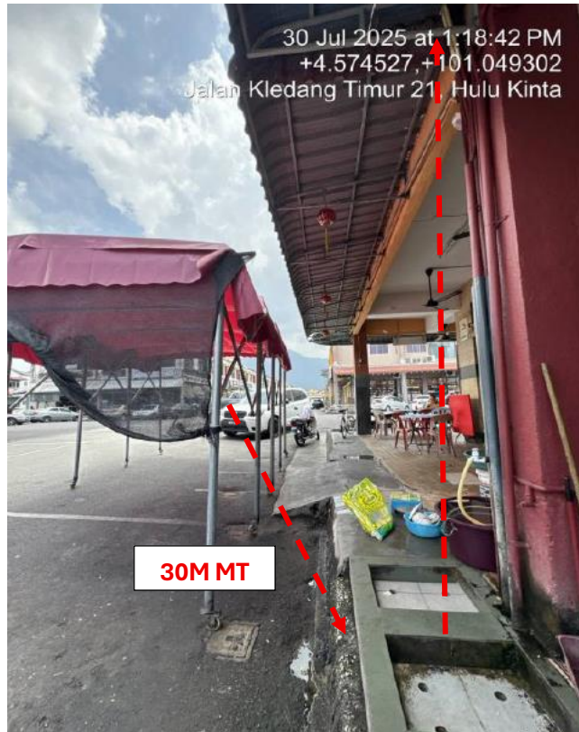
PICTURE 5 : MICROTRENCHING 30M TO CABINET BUILDING
