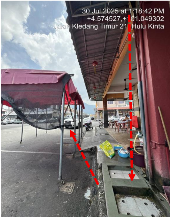
Picture 7 – TRENCHING 30M TO PROPOSE MH
