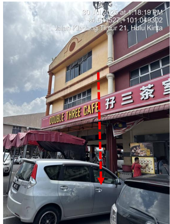
Picture 6 – TRUNKING AND GI PIPE 30M
