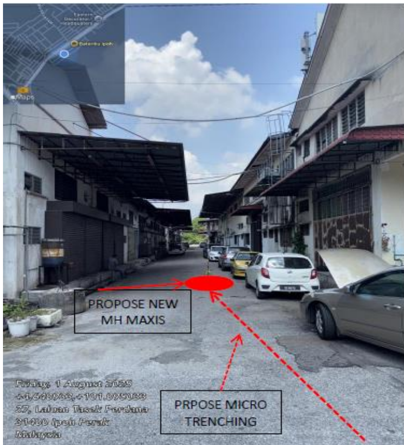
PICTURE 2 : PROPOSE 70M MICROTRENCHING TO PROP MH01
