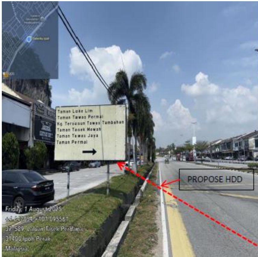
PICTURE 3 : PROPOSE 160M HDD WORK TO PROP MH01
