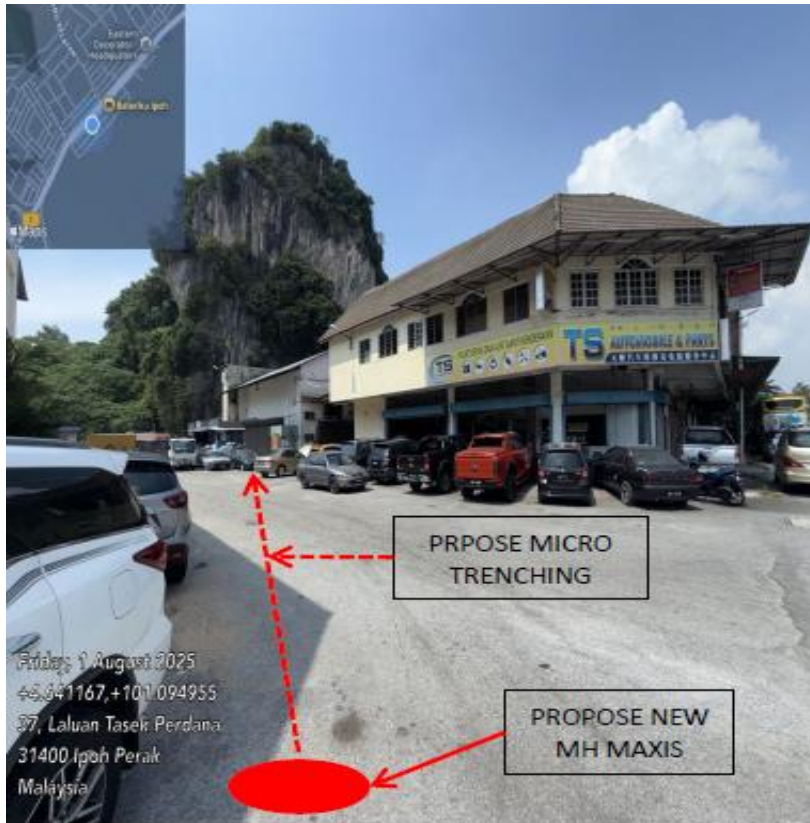
PICTURE 5 : PROPOSE 70M MICROTRENCHING TO PROP MH02
