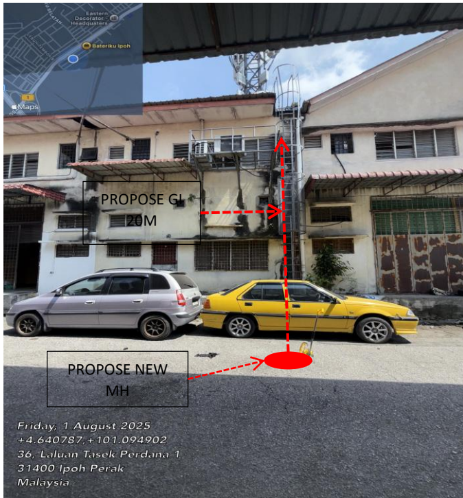
Picture 8 - PROPOSE NEW HDD WORK TOWARDS UM SITE
