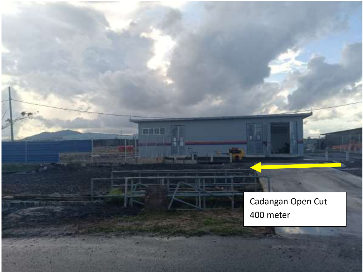
Gambar 13 : Pencawang Baru (Greenverse Substation)
