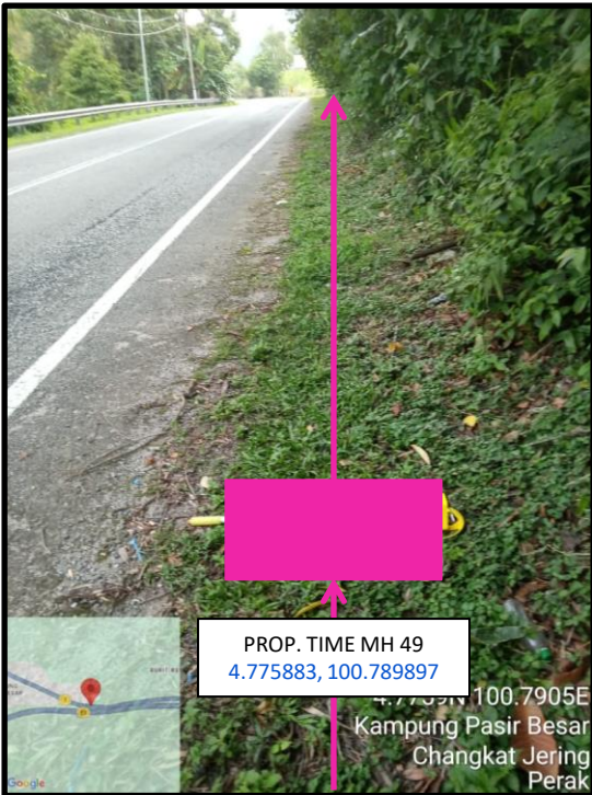
Proposed HDD 1 Way and Pulling Cable 144C from Prop. TIME MH49 to Prop. TIME MH50 at Kampung Pasir Besar
