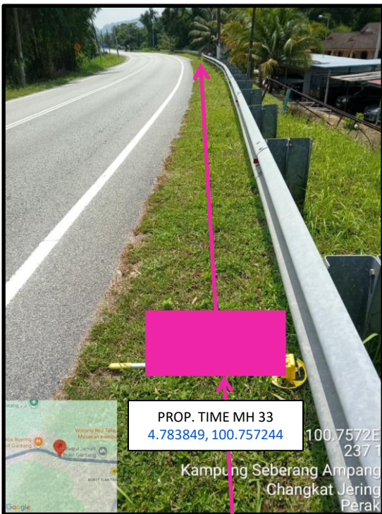
Proposed HDD 1 Way and Pulling Cable 144C from Prop. TIME MH33 to Prop. TIME MH34 at Bukit Gantang
