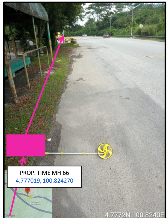
Proposed HDD 1 Way and Pulling Cable 144C from Prop. TIME MH66 to Prop. TIME MH67 at beside the highway
