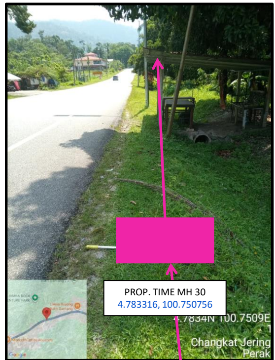
Proposed HDD 1 Way and Pulling Cable 144C from Prop. TIME MH30 to Prop. TIME MH31 at Changkat Jering
