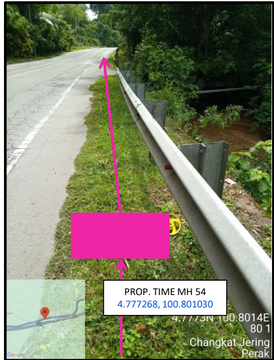
Proposed HDD 1 Way and Pulling Cable 144C from Prop. TIME MH54 to Prop. TIME MH55 at beside the highway
