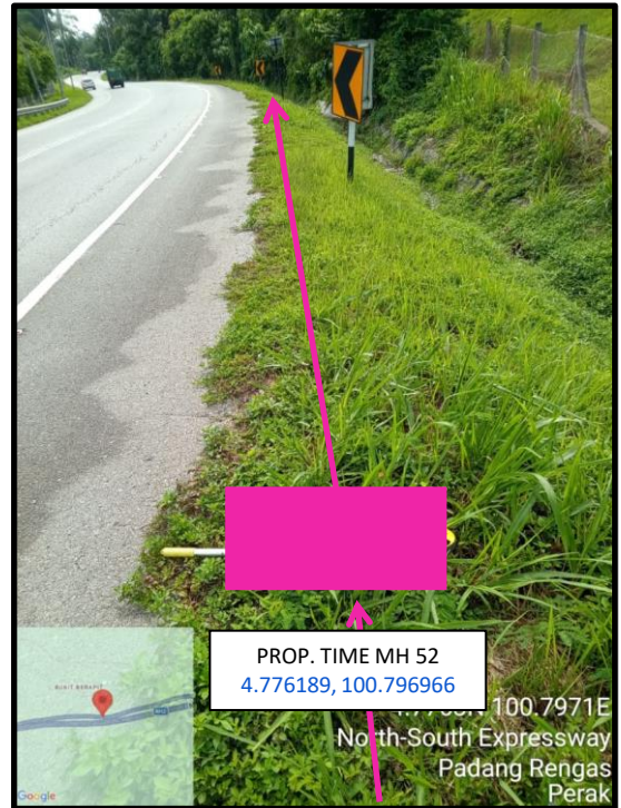
Proposed HDD 1 Way and Pulling Cable 144C from Prop. TIME MH52 to Prop. TIME MH53 at beside the highway
