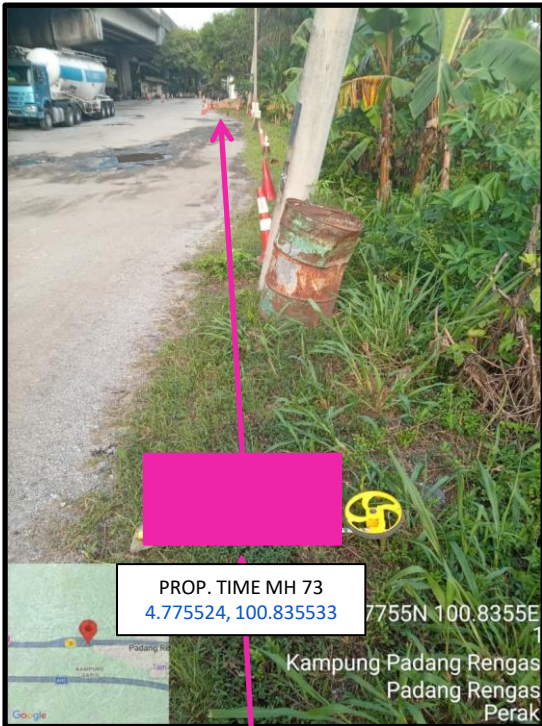
Proposed HDD 1 Way and Pulling Cable 144C from Prop. TIME MH73 to Prop. TIME MH74 at Kampung Padang Rengas
