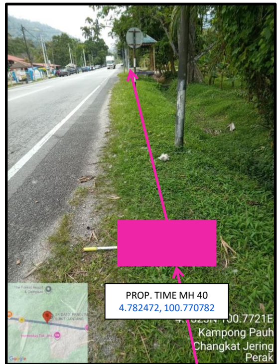
Proposed HDD 1 Way and Pulling Cable 144C from Prop. TIME MH40 to Prop. TIME MH41 at Kampung Pasir Besar
