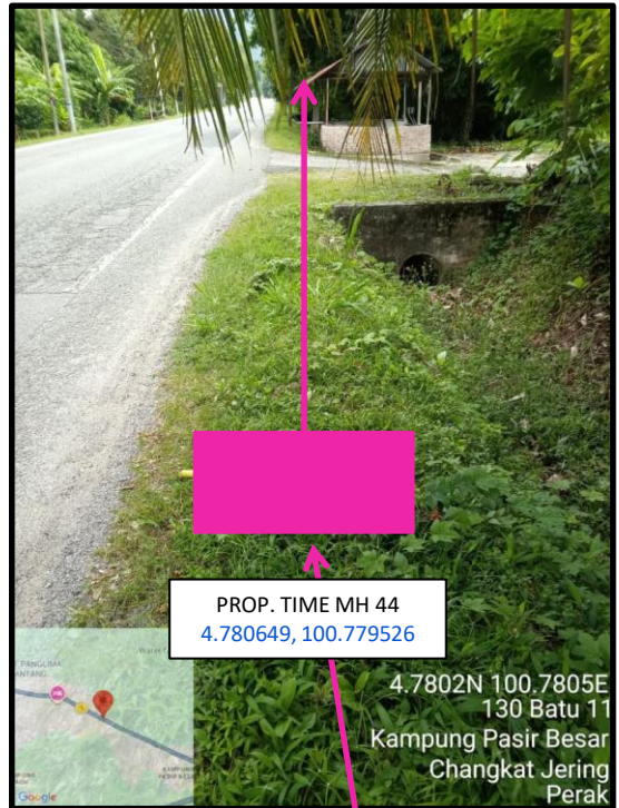
Proposed HDD 1 Way and Pulling Cable 144C from Prop. TIME MH44 to Prop. TIME MH46 at Kampung Pasir Besar
