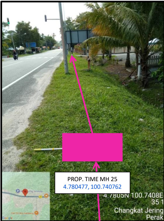
Proposed HDD 1 Way and Pulling Cable 144C from Prop. TIME MH25 to Prop. TIME MH26 at Jalan Enam Kaki
