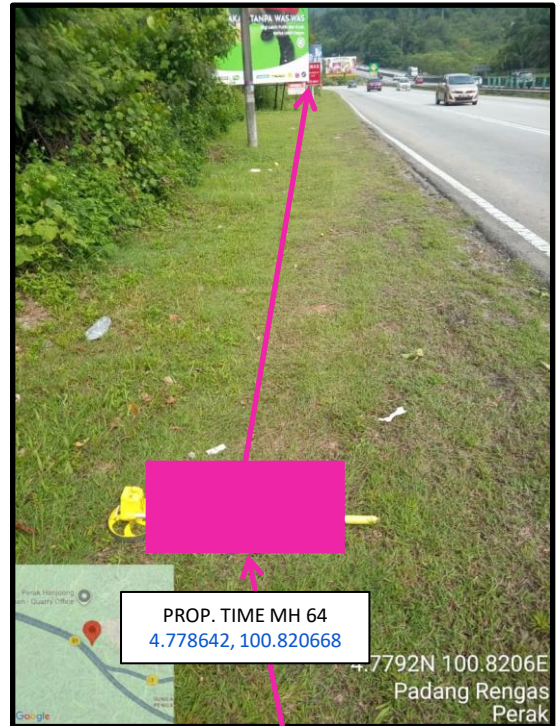
Proposed HDD 1 Way and Pulling Cable 144C from Prop. TIME MH64 to Prop. TIME MH65 at beside the highway
