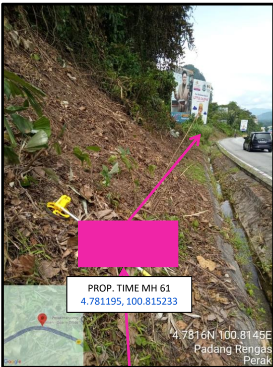
Proposed HDD 1 Way and Pulling Cable 144C from Prop. TIME MH61 to Prop. TIME MH62 at beside the highway
