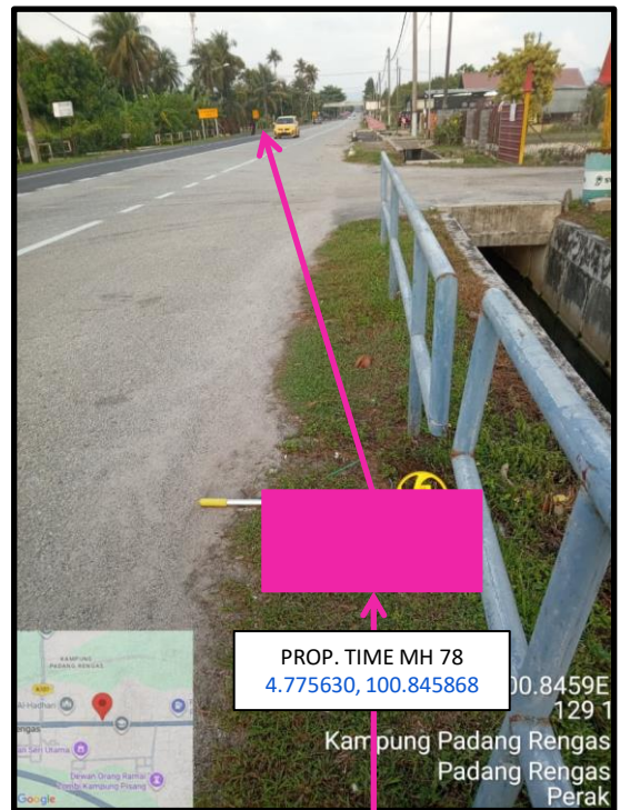
Proposed HDD 1 Way and Pulling Cable 144C from Prop. TIME MH78 to Prop. TIME MH79 at Kampung Padang Rengas
