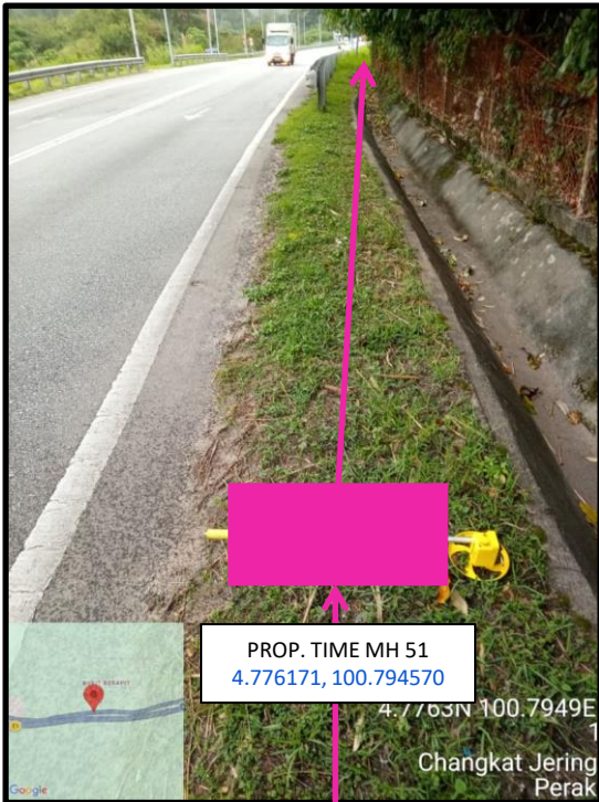
Proposed HDD 1 Way and Pulling Cable 144C from Prop. TIME MH51 to Prop. TIME MH52 at beside the highway
