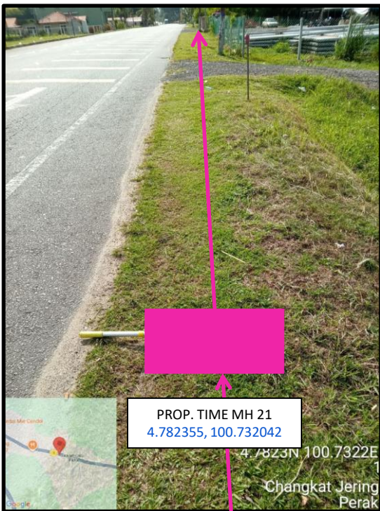
Proposed HDD 1 Way and Pulling Cable 144C from Prop. TIME MH21 to Prop. TIME MH22 at Jalan Enam Kaki
