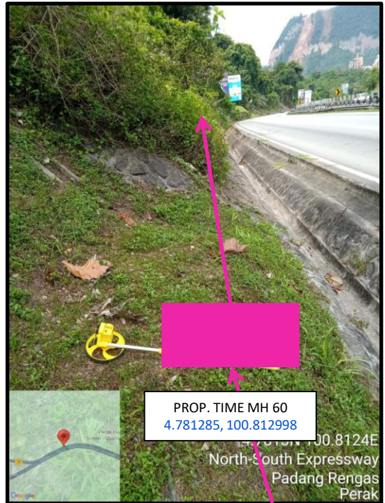
Proposed HDD 1 Way and Pulling Cable 144C from Prop. TIME MH60 to Prop. TIME MH61 at Kampung Pasir Besar
