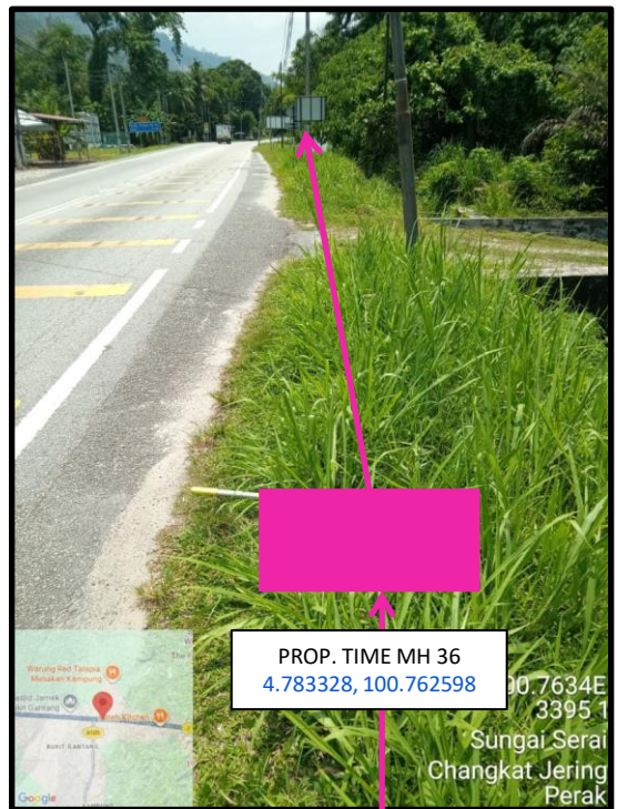
Proposed HDD 1 Way and Pulling Cable 144C from Prop. TIME MH36 to Prop. TIME MH37 at Bukit Gantang
