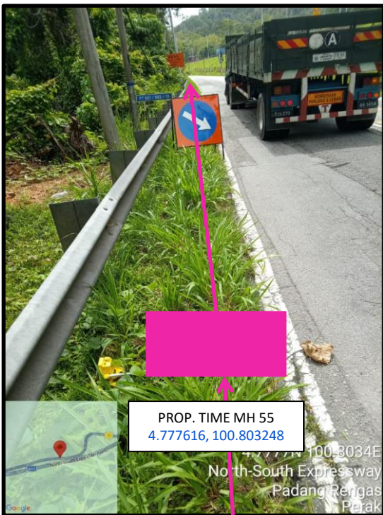
Proposed HDD 1 Way and Pulling Cable 144C from Prop. TIME MH55 to Prop. TIME MH56 at beside the highway
