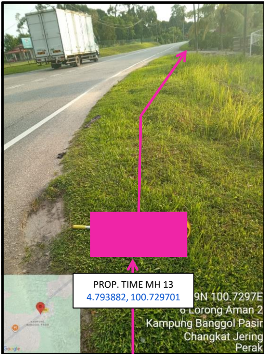
Proposed HDD 1 Way and Pulling Cable 144C from Prop. TIME MH13 to Prop. TIME MH14 at Lorong Aman 2
