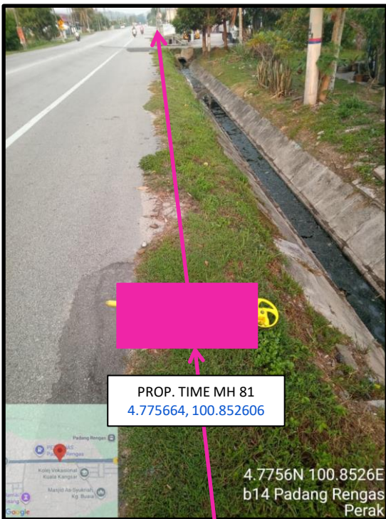
Proposed HDD 1 Way and Pulling Cable 144C from Prop. TIME MH81 to Prop. TIME MH82 at Taman Seri Permai
