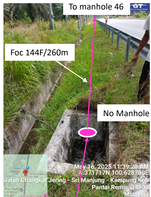
Manhole 45 Way blockage to MH 46, Cable on pole, Manhole need to raise up. Prop New HDD Mh 45 to Mh 46
