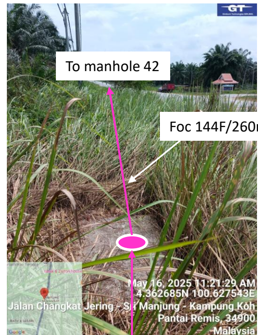
Manhole 41 Way ok Mh 42 to Mh 41
