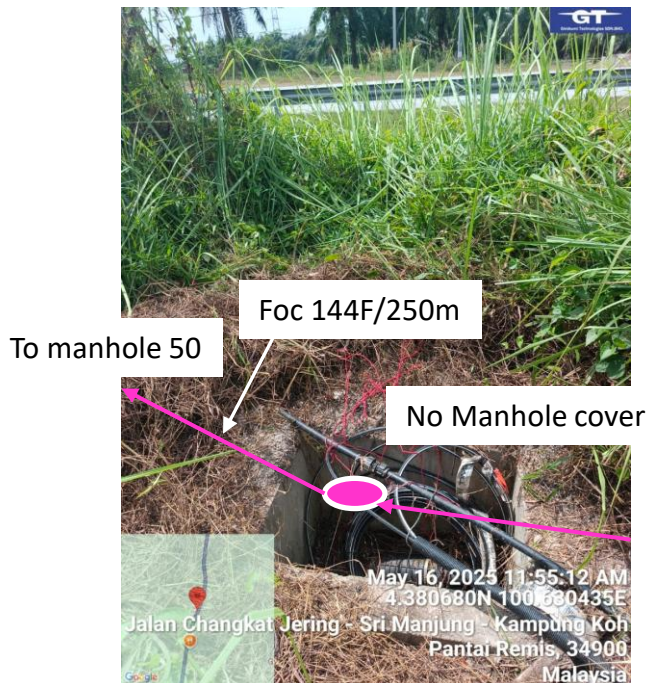
Manhole 49 Way ok Mh 49 to Mh 50
