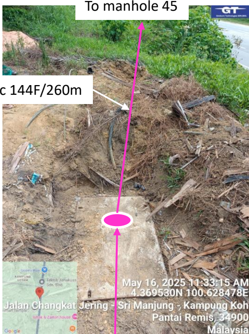
Manhole 44 Manhole need to raise up Way ok Mh 45 to Mh 44
