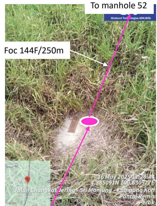
Manhole 51 Way ok Mh 52 to Mh 51,
