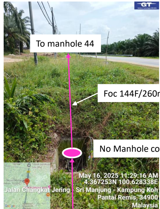
Manhole 43 Manhole need to raise up Way ok Mh 44 to Mh 43
