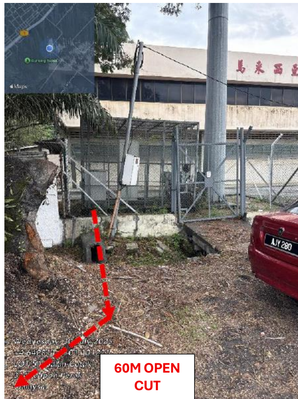
PICTURE 1 : PROPOSE OPEN TRENCH
