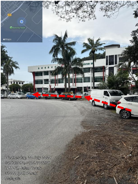
Picture 5 – PROPOSE OPEN TRENCH ON GRASS VERGE TO EXISTING MAXIS MH
