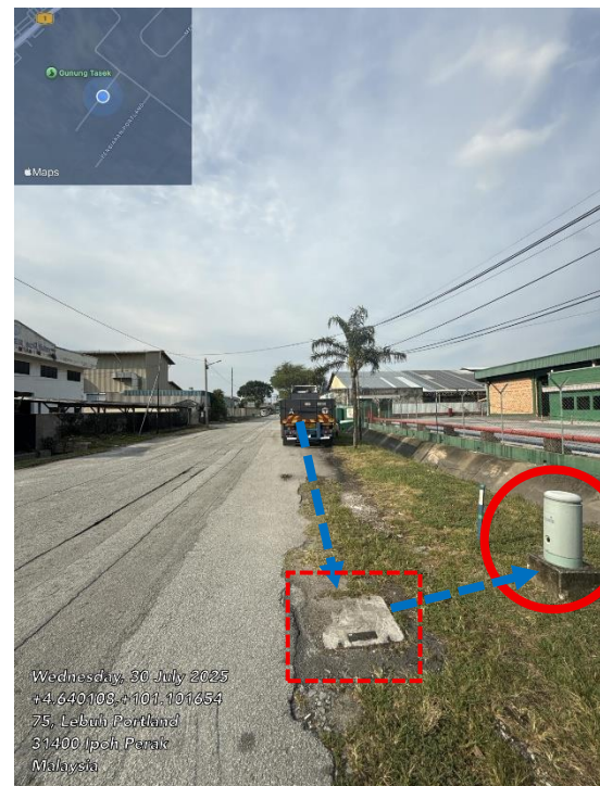
Picture 8 – PROPOSE NEW CABLE IN EXISTING WAY. TAPPING TO MAXIS FDP
