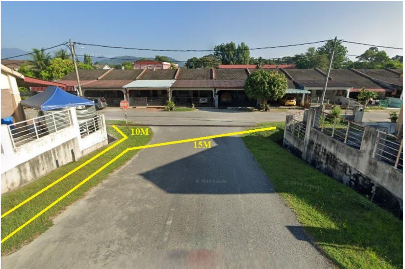
GAMBAR 1 : CAD CUT AND JOINT UG KABEL HT KLPE 150MMP KE P/E TAMAN SENTOSA
