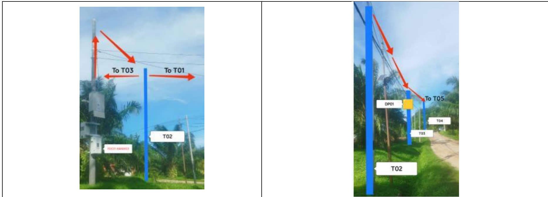
Site Photos – Proposed to install pole 7.5m
