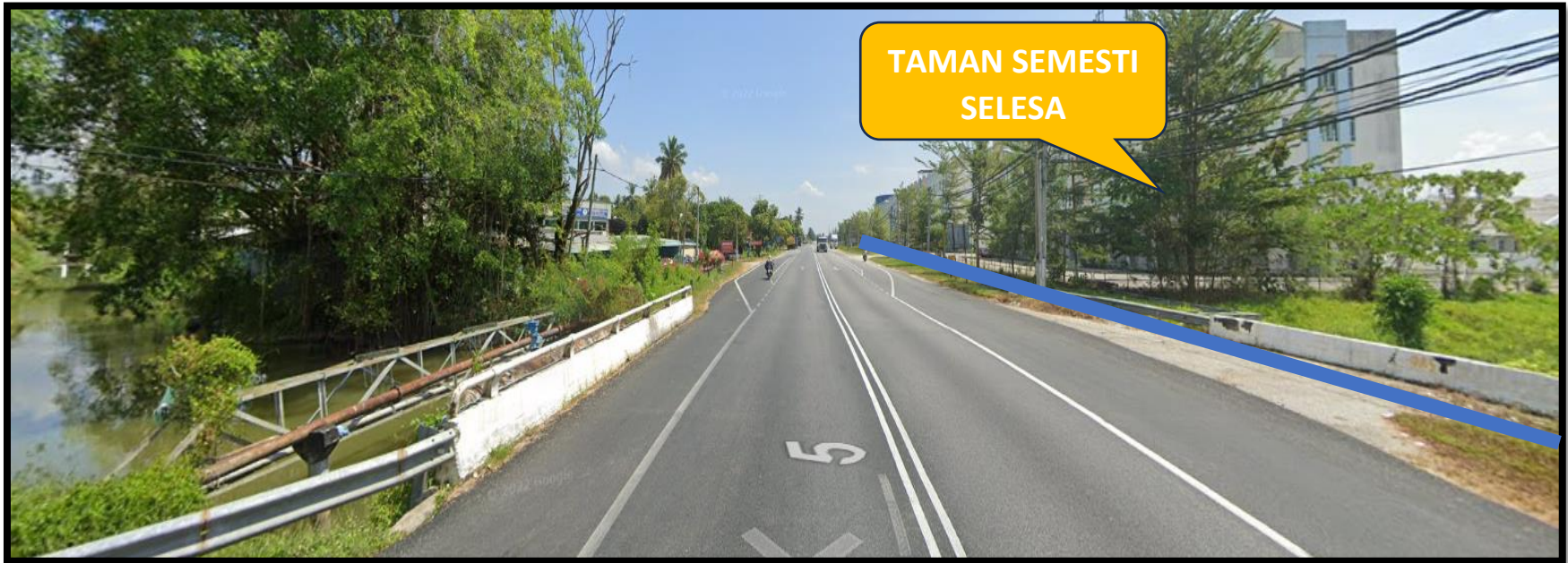
FIGURE 1.6: JALAN KLANG – TELUK INTAN (5)
