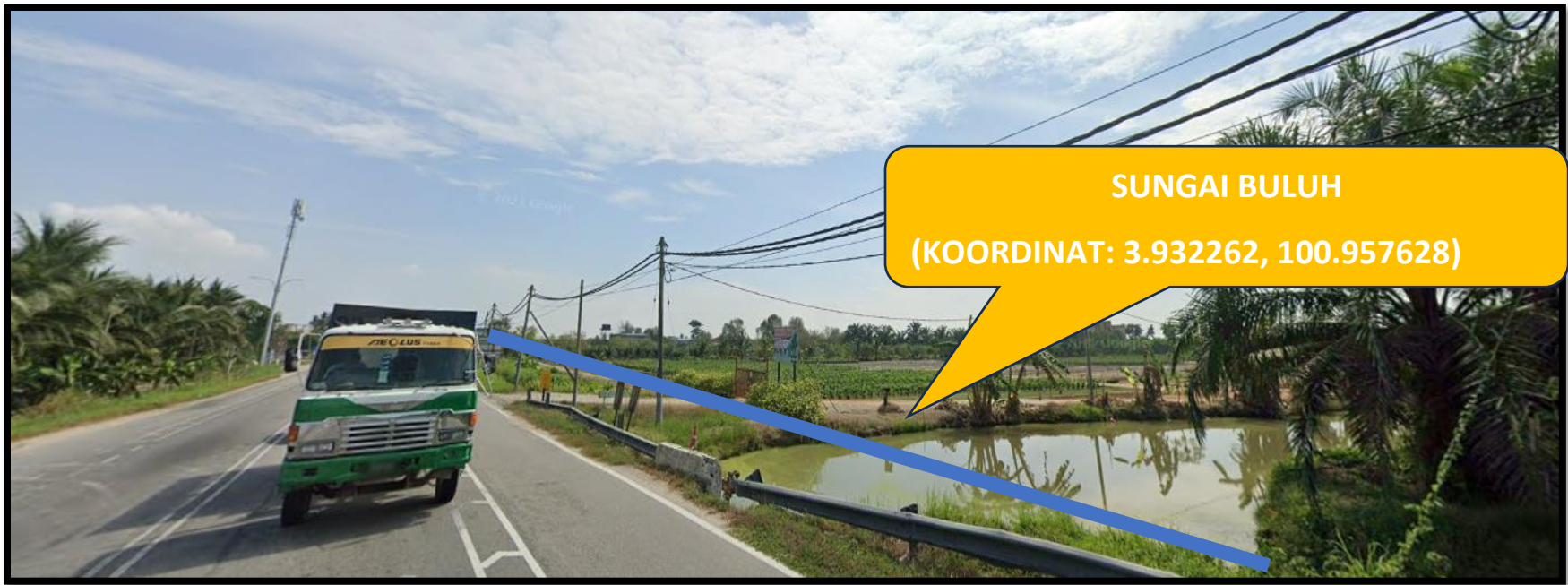
FIGURE 1.4: JALAN KLANG – TELUK INTAN (5)
