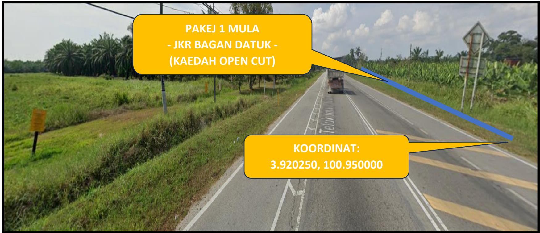
FIGURE 1.1: JALAN KLANG – TELUK INTAN (5)
