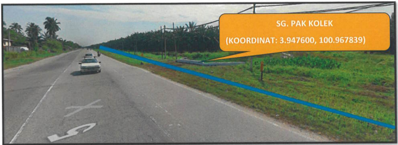
FIGURE 1.7: JALAN KLANG – TELUK INTAN (5)
