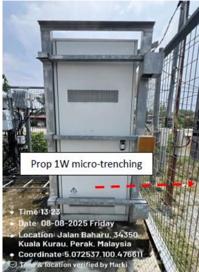
PICTURE 3 : PROPOSE MICROTRENCHING TO UM CABINET
