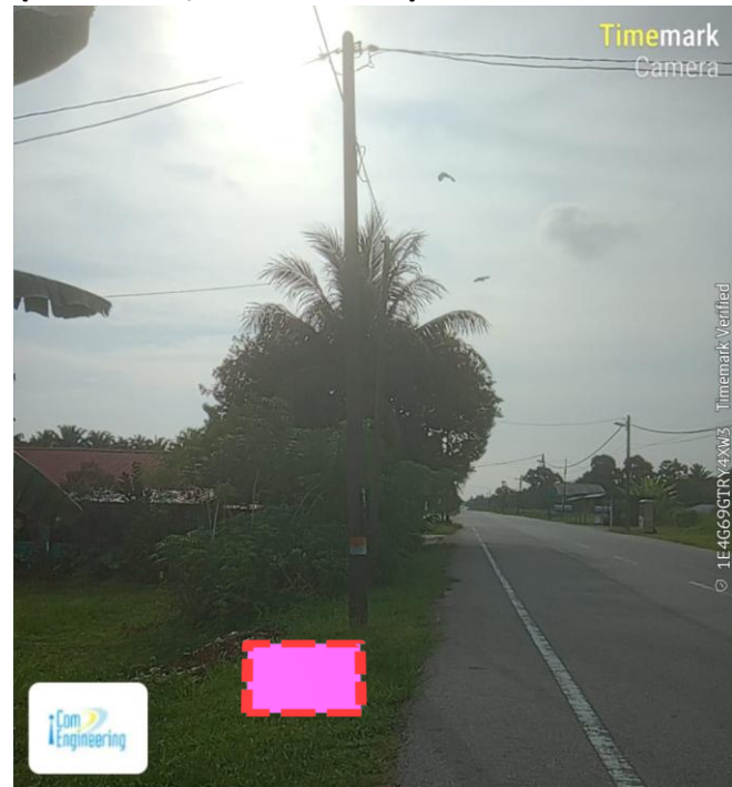
Prop New TIME MH 23 (Jalan Labu Kubong) (4.127581, 101.110604)
