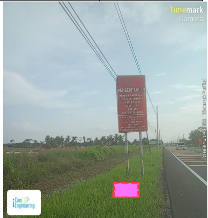
Prop New TIME MH 57 (Jalan Labu Kubong) (4.099158, 101.049405)
