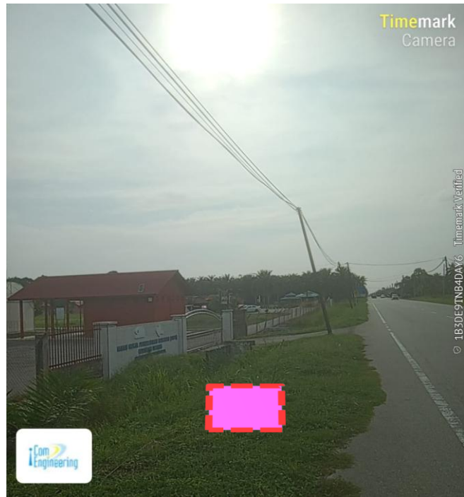
Prop New TIME MH 17 (Jalan Labu Kubong) (4.121295, 101.122018)
