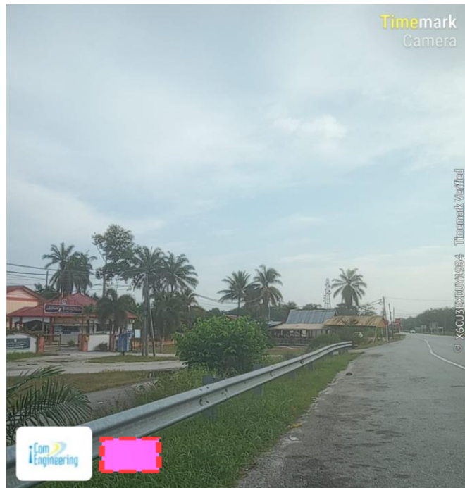
Prop New TIME MH 31 (Jalan Labu Kubong) (4.131933, 101.095613)
