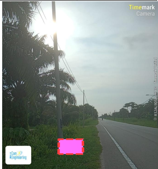
Prop New TIME MH 25 (Jalan Labu Kubong) (4.129595, 101.106772)
