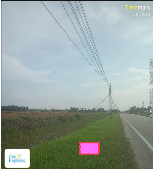
Prop New TIME MH 56 (Jalan Labu Kubong) (4.100251, 101.051199)
