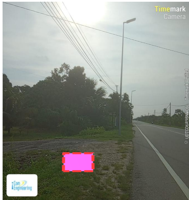
Prop New TIME MH 19 (Jalan Labu Kubong) (4.123335, 101.118205)
