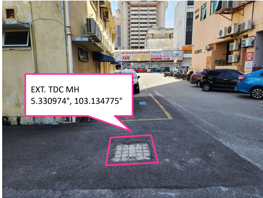
Existing TDC Manhole (Pro. Joint MH)
