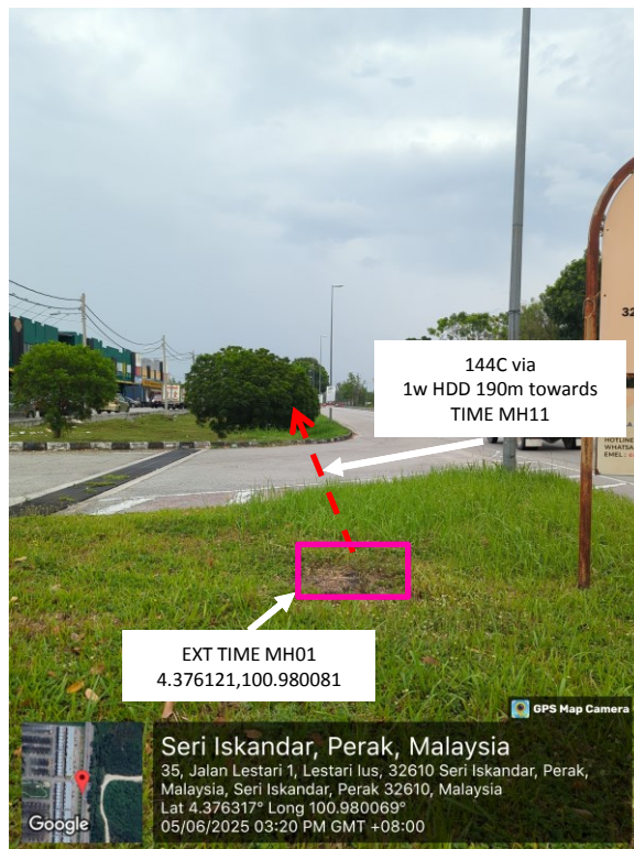
Existing TIME MH01 and prop 1w HDD to TIME MH11 at Ipoh – Lumut Highway (JKR)
