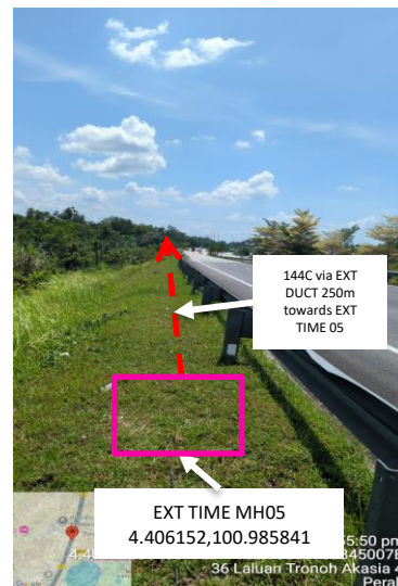
Existing TIME MH05 and prop 144C Cable pulling via EXT Duct to EXT TIME MH06 at Ipoh – Lumut Highway (JKR)
