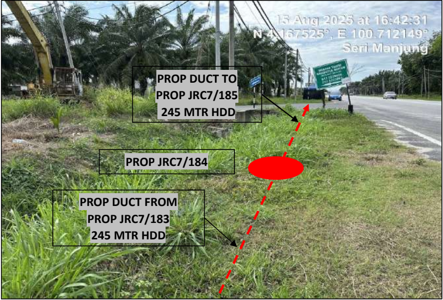
LOCATION AT JALAN (5)
