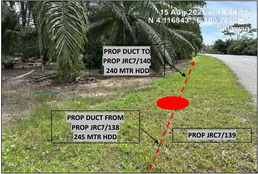
LOCATION AT JALAN (5)
