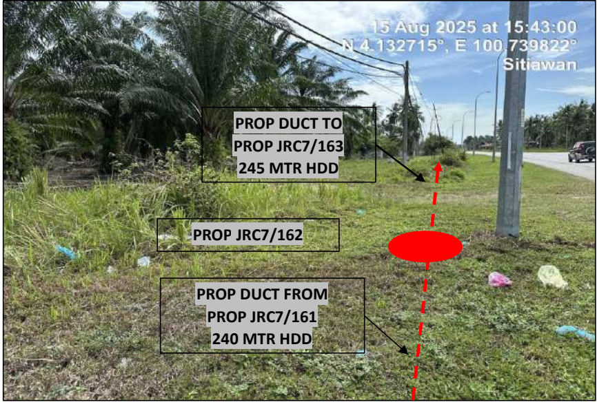
LOCATION AT JALAN (5)
