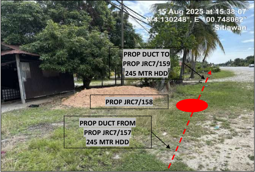
LOCATION AT JALAN (5)
