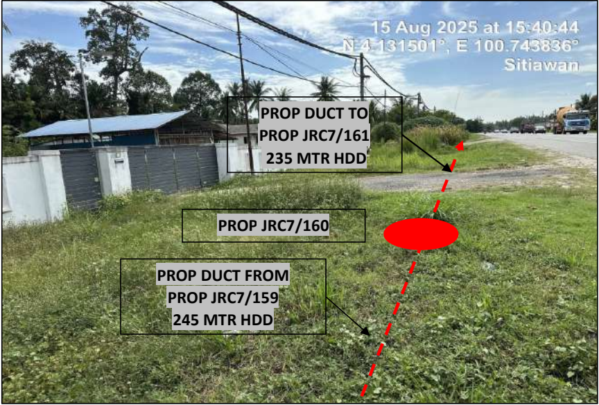
LOCATION AT JALAN (5)
