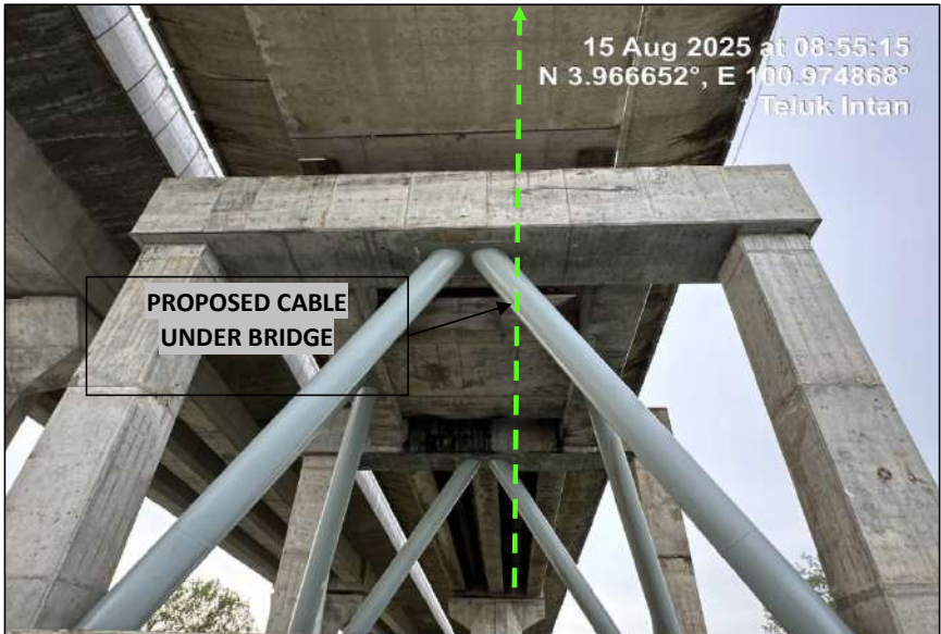
LOCATION AT JAMBATAN SUNGAI PERAK
