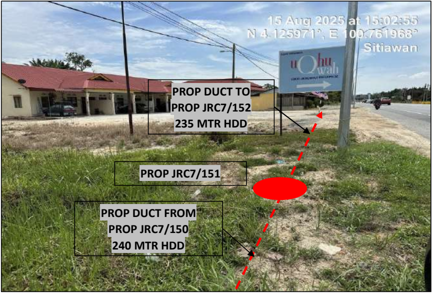
LOCATION AT JALAN (5)
