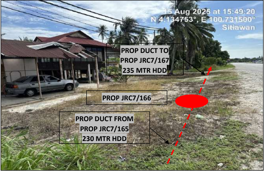
LOCATION AT JALAN (5)
