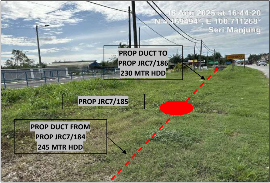
LOCATION AT JALAN (5)
