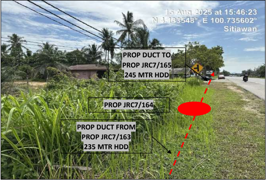
LOCATION AT JALAN (5)
