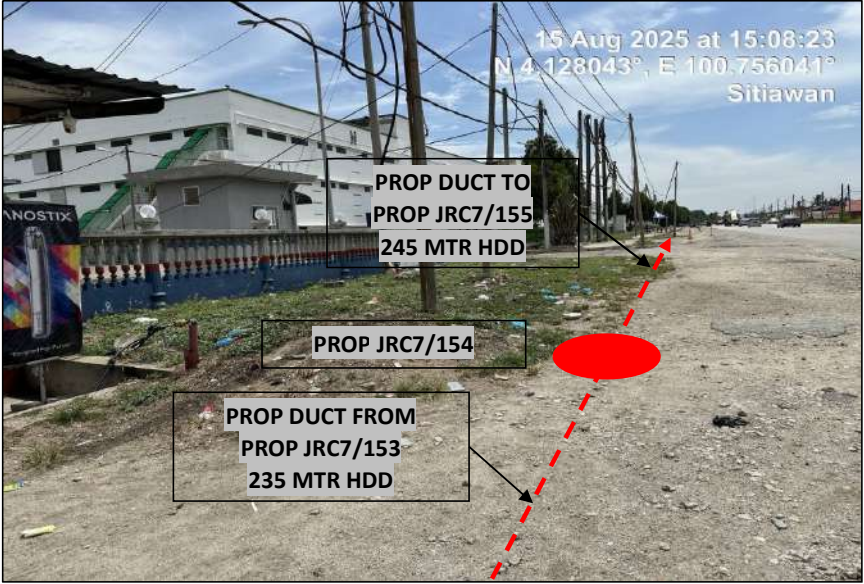
LOCATION AT JALAN (5)
