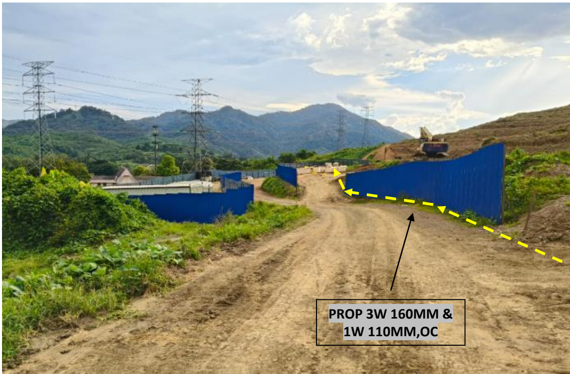
LOCATION AT PRIVATE ROAD
