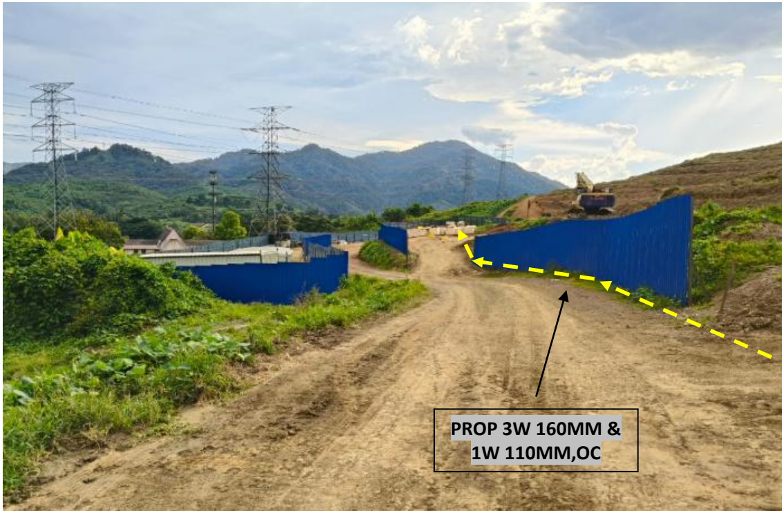
LOCATION AT PRIVATE ROAD
