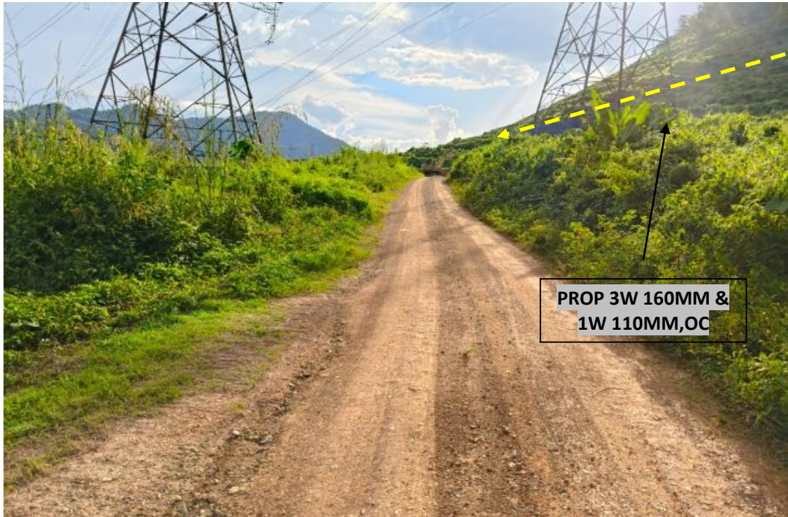
LOCATION AT PRIVATE ROAD
