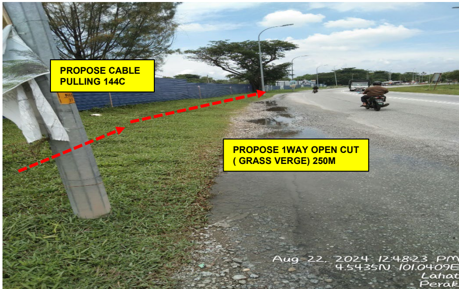
LOCATION : JALAN LAHAT
