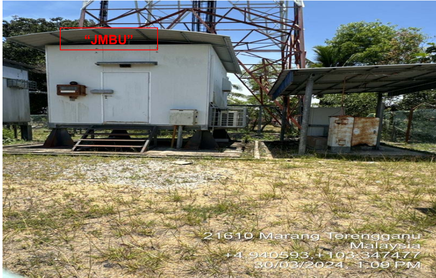
LOCATION AT "JMBU"
