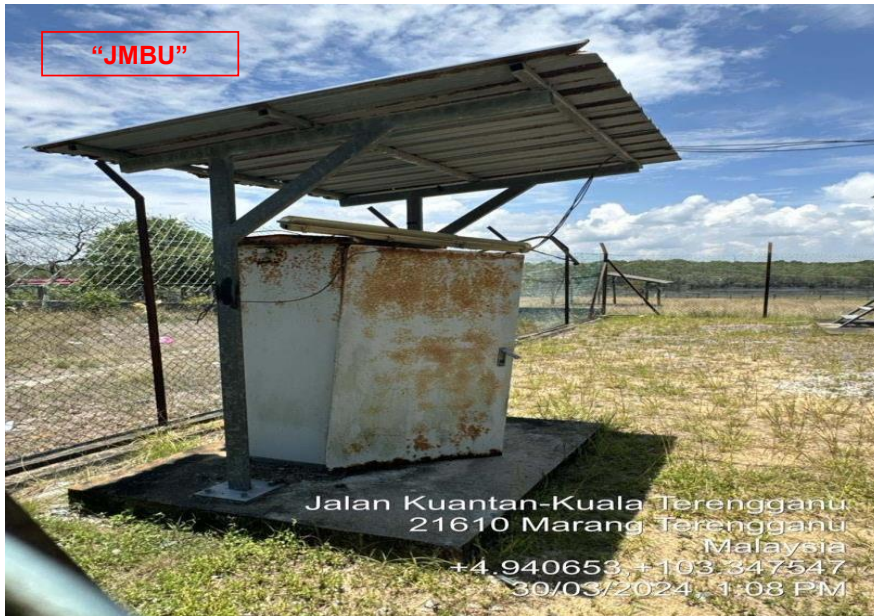
LOCATION AT "JMBU"
