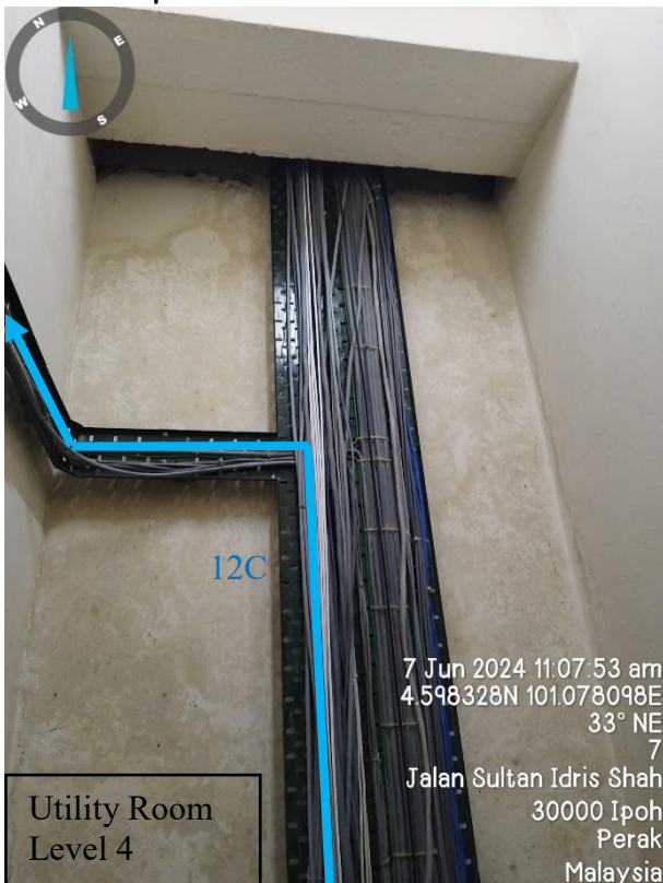
Propose cable pulling
