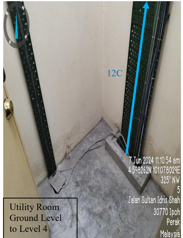
Propose cable pulling
