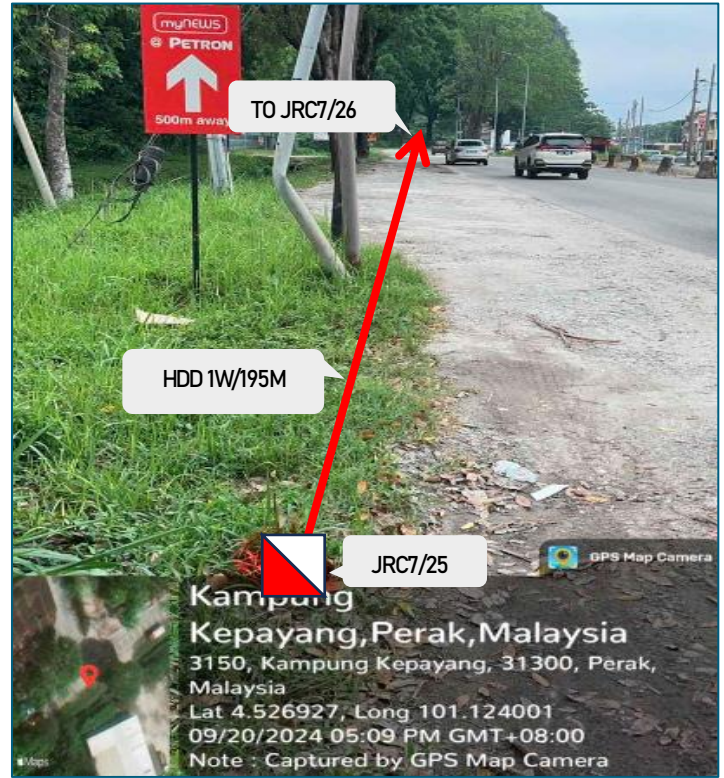
PROP JRC7/25 AT JLN SIMPANG PULAI-LAHAT (ROADSIDE)
