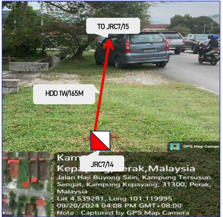
PROP JRC7/14 AT JLN HAJI BUYONG SILIN (ROADSIDE)
