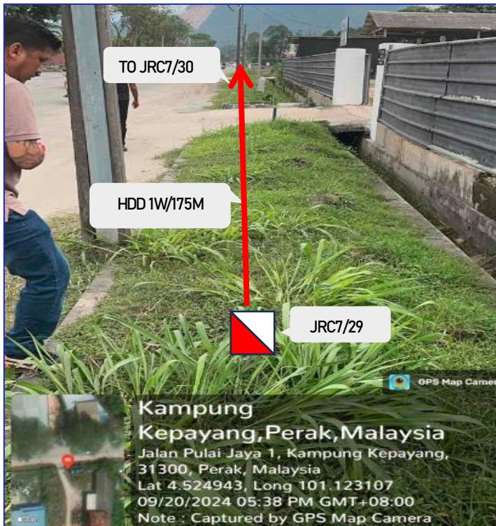
PROP JRC7/29 AT JALAN PULAI JAYA 1 (ROADSIDE)
