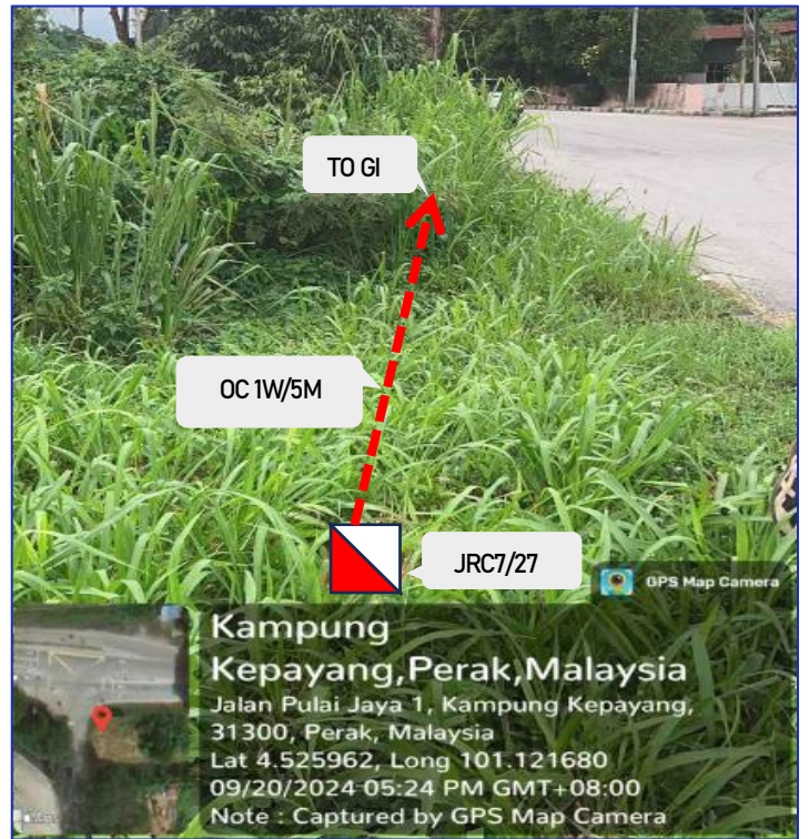
PROP JRC7/27 AT JLN SIMPANG PULAI-LAHAT (ROADSIDE)
