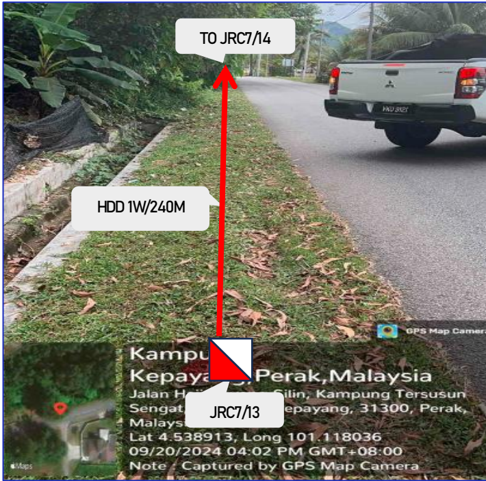
PROP JRC7/13 AT JLN HAJI BUYONG SILIN (ROADSIDE)
