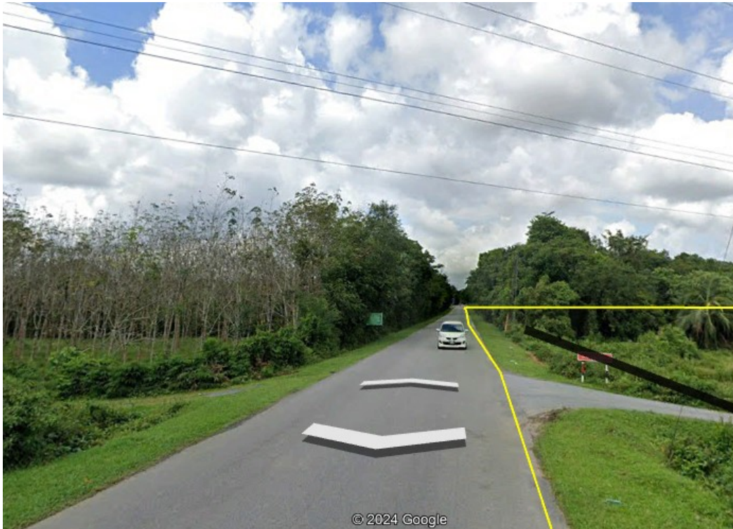
Open Cut 2: TNB Pylon
