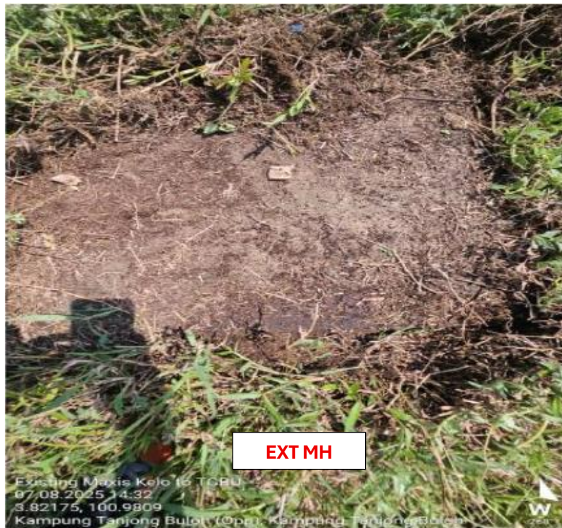
PICTURE 1 : EXISTING MAXIS MANHOLE
