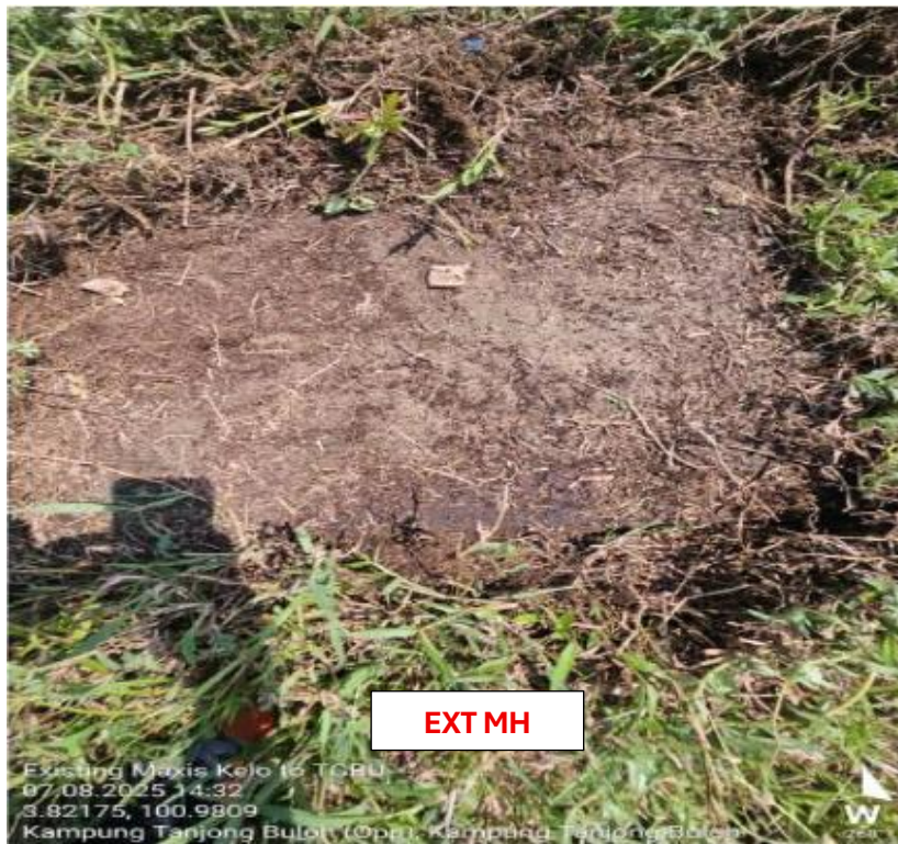
PICTURE 1 : EXISTING MAXIS MANHOLE
