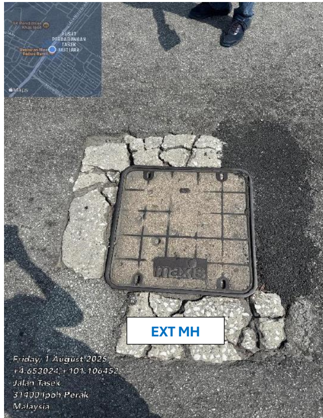
PICTURE 1 : EXISTING MANHOLE
