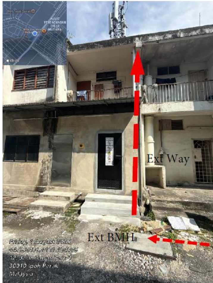
PICTURE 3 : BUILDING MANHOLE
