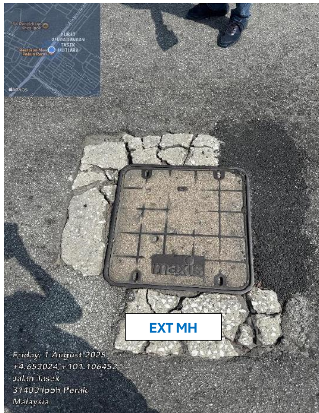
PICTURE 1 : EXISTING MANHOLE
