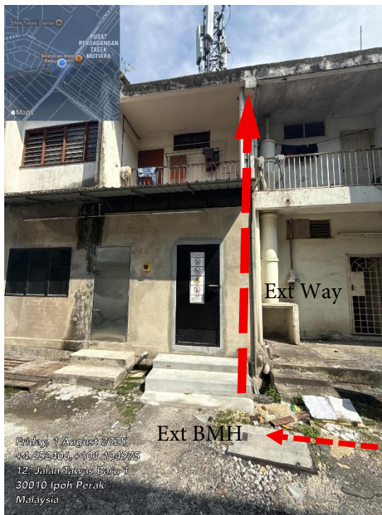
Picture 3 – HDD towards Ext BMH
