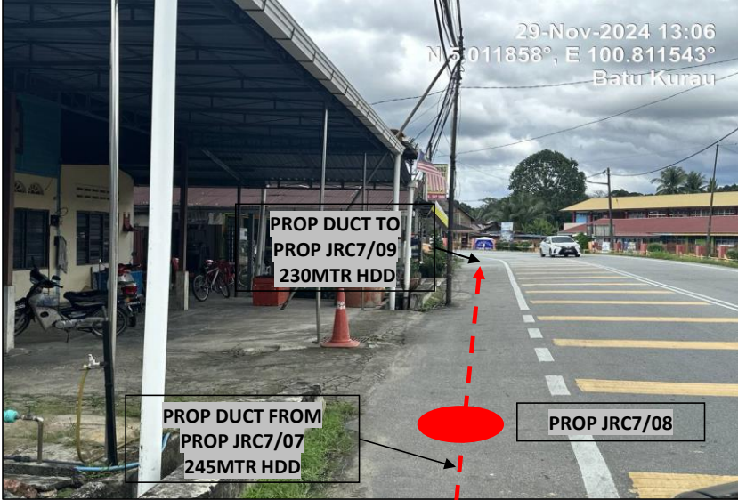
LOCATION AT JALAN (A5)
