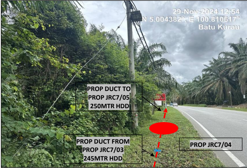
LOCATION AT JALAN (A5)
