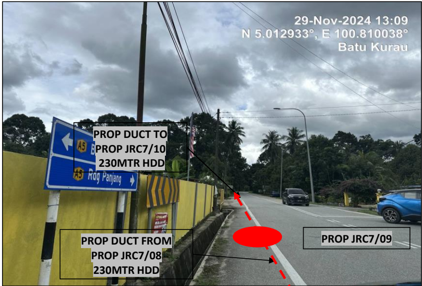
LOCATION AT JALAN (A5)
