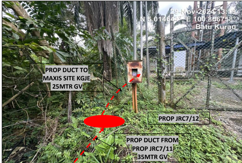
LOCATION AT MAXIS SITE KGJE
