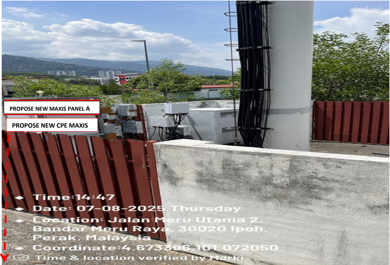
PICTURE 1 : PROPOSE ONE (1) MAXIS EQUIPMENT AND ONE (1) MAXIS PANEL A AT UM T5.
