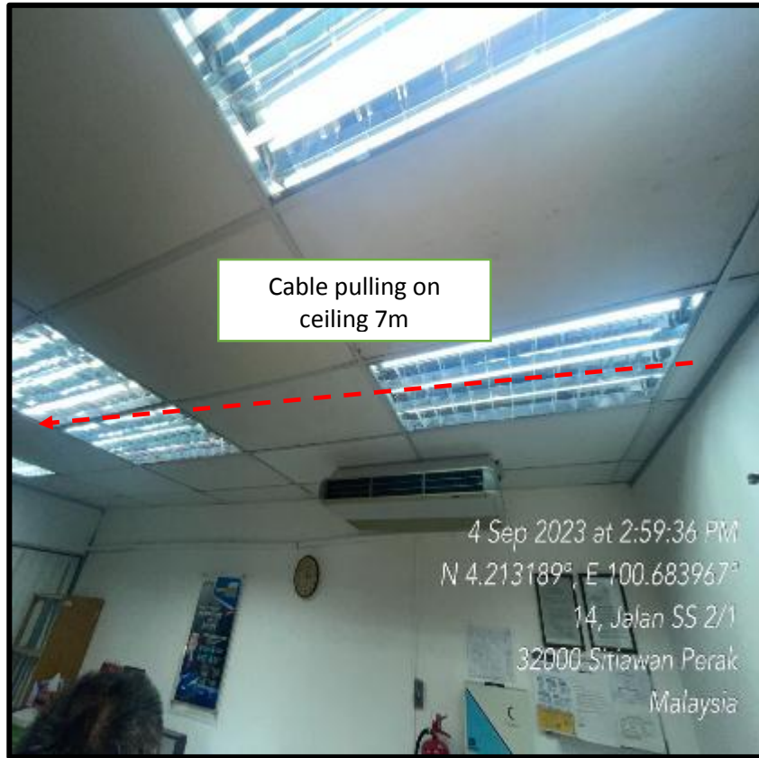
Cable 48c pulling on Ceiling at Main Office room
