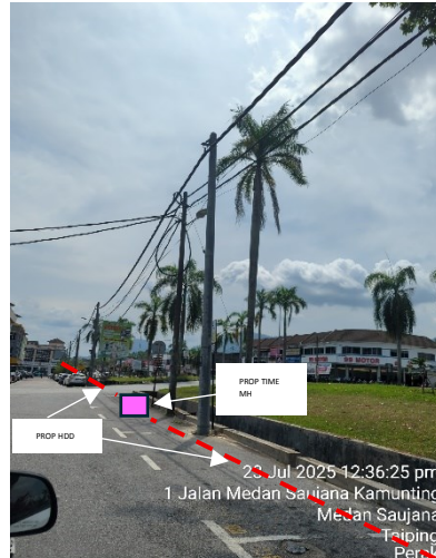
PROP HDD and TIME MH AT JALAN KAMUNTING
