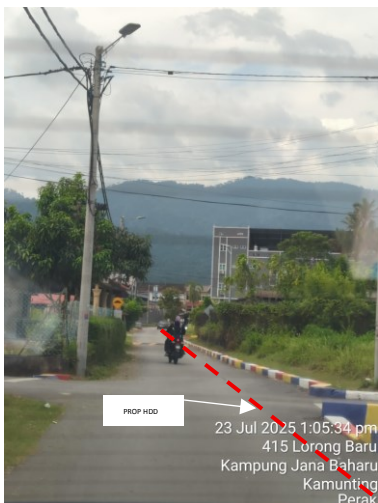
PROP HDD AT JALAN LAMA
