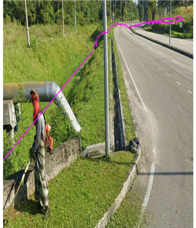
JALAN IPOH - KAMPAR (OPEN CUT)
