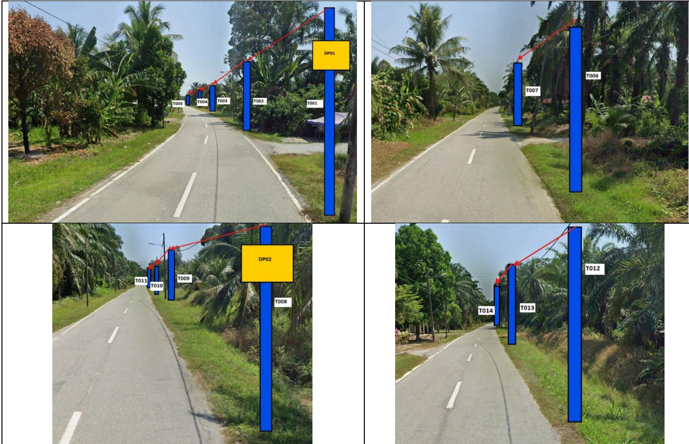
Site Photos – Proposed to install pole 7.5m
