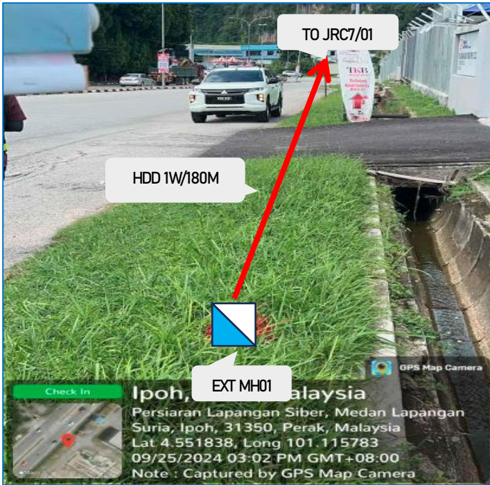
EXT MH01 AT JALAN PESIARAN SIBER 1 (ROADSIDE)
