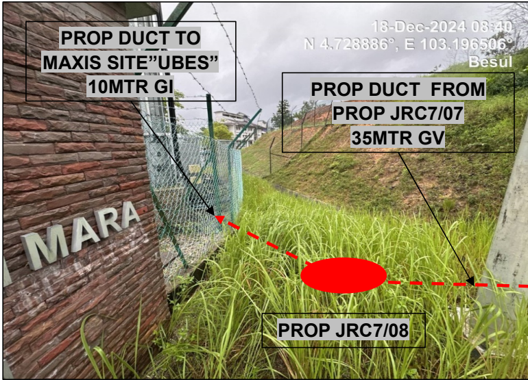
LOCATION AT MAXIS SITE "UBES"
