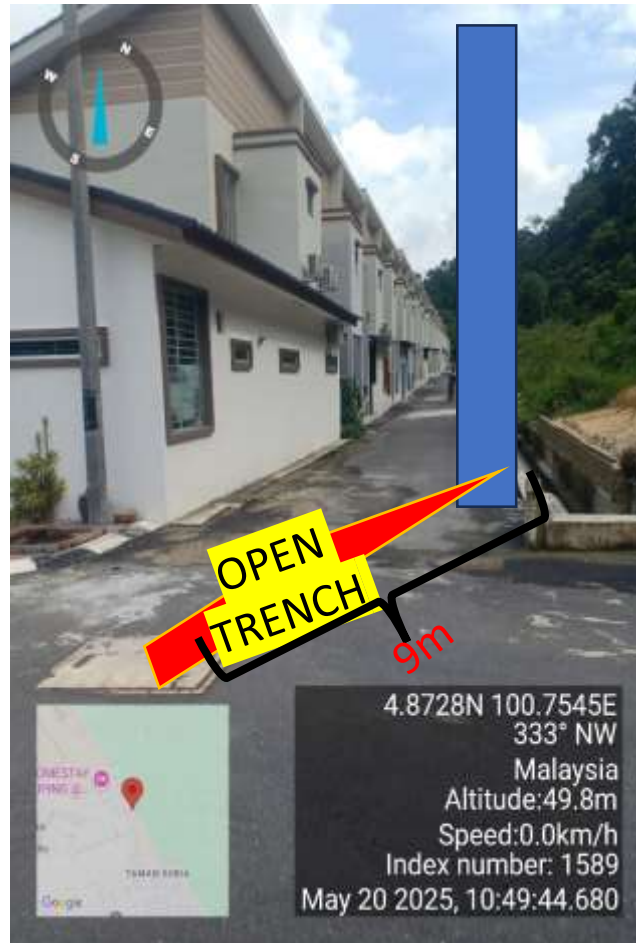
TRENCHING FROM MH TO POLE 1
