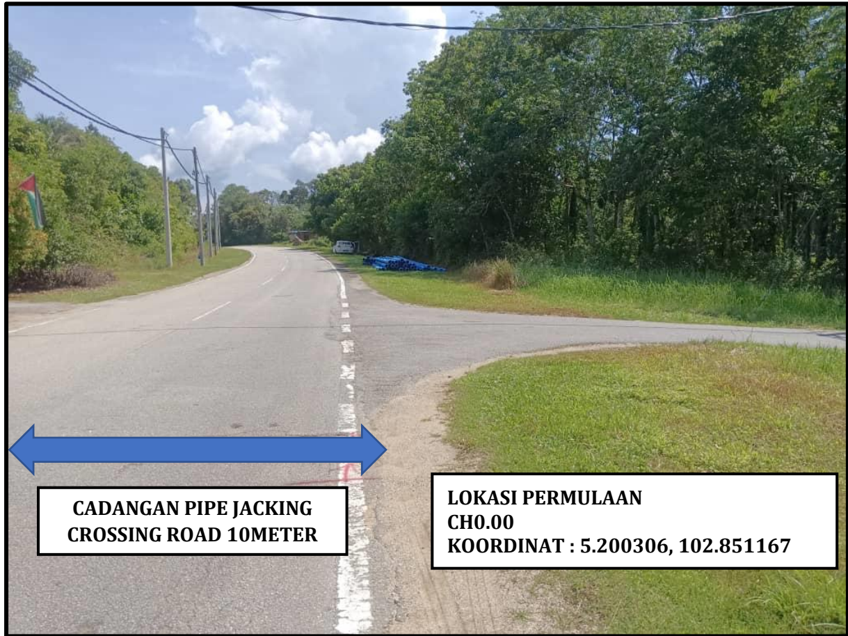
GAMBAR 1 : CH0.00 PERMULAAN KERJA PIPE JACKING CROSSING ROAD
