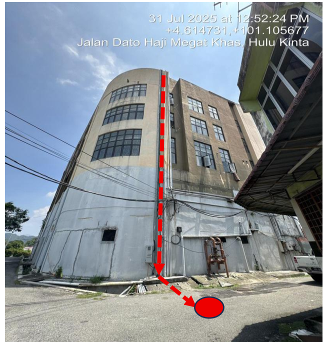
Picture 4 – CABLE WAY TRUNKING AND TRENCING
