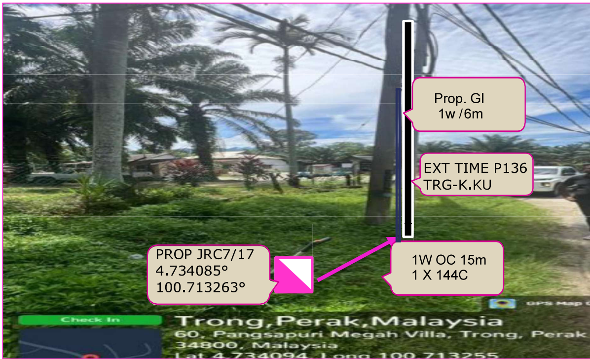
PROP 144C CABLE ROUTING VIA PROP JRC7/17 AT JALAN BESAR (ROADSIDE)
