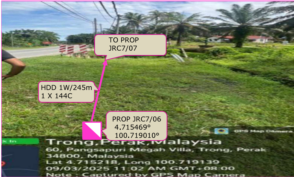
PROP 144C CABLE ROUTING VIA PROP JRC7/06 AT JALAN BESAR (ROADSIDE)
