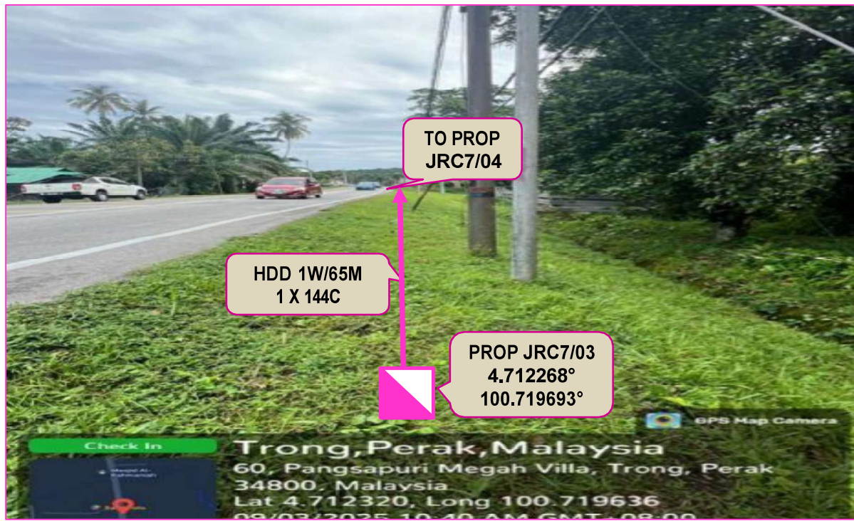
PROP 144C CABLE ROUTING VIA PROP JRC7/03 AT JALAN BESAR (ROADSIDE)
