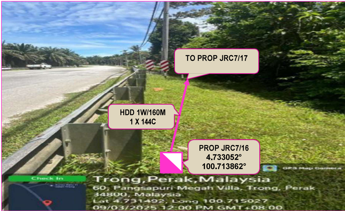
PROP 144C CABLE ROUTING VIA PROP JRC7/16 AT JALAN BESAR (ROADSIDE)
