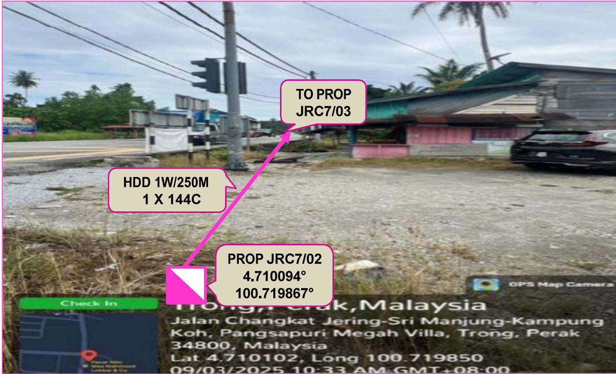
PROP 144C CABLE ROUTING VIA PROP JRC7/02 AT JALAN BESAR (ROADSIDE)
