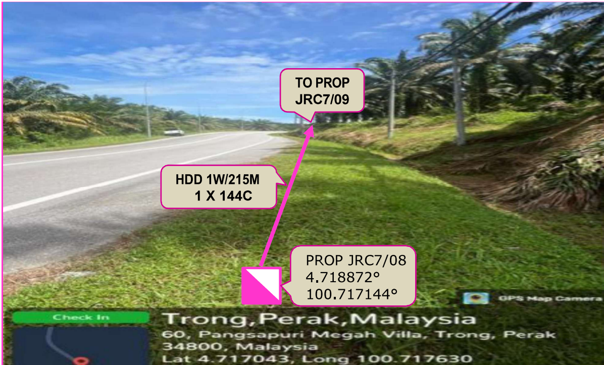
PROP 144C CABLE ROUTING VIA PROP JRC7/08 AT JALAN BESAR (ROADSIDE)
