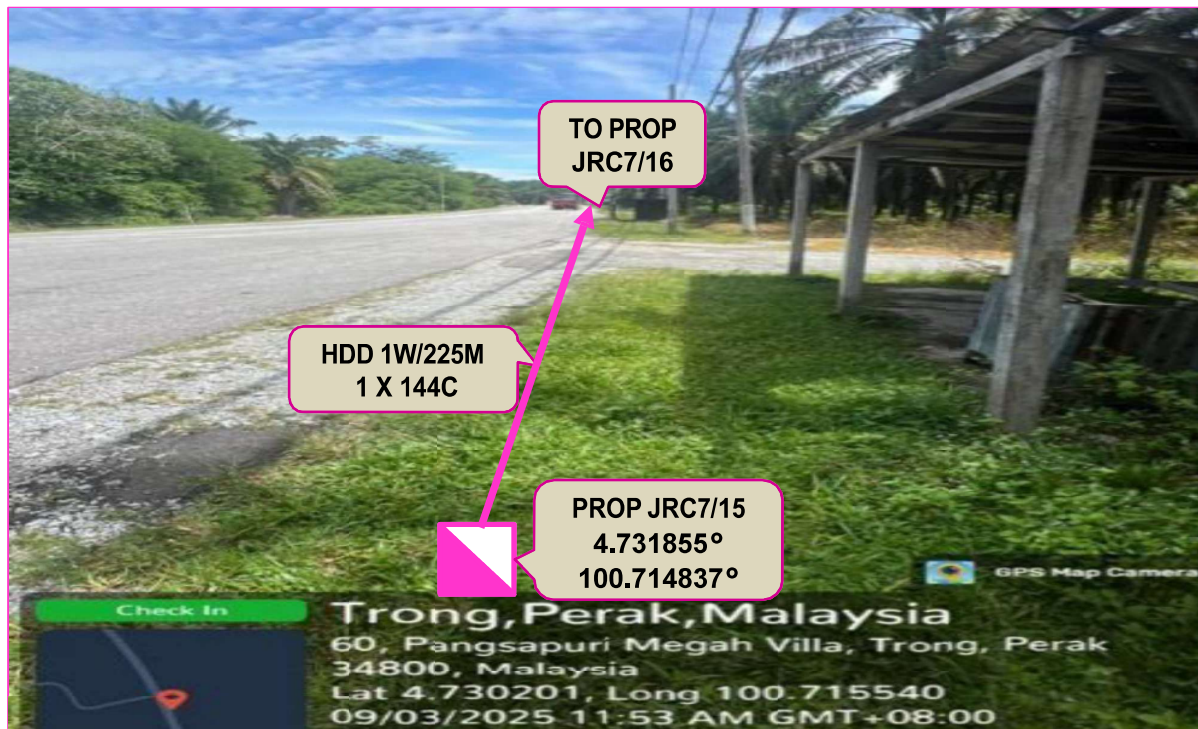
PROP 144C CABLE ROUTING VIA PROP JRC7/15 AT JALAN BESAR (ROADSIDE)
