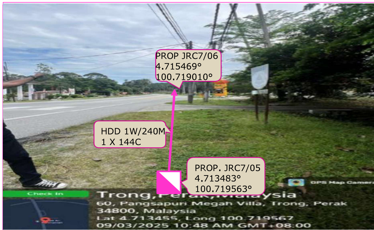
PROP 144C CABLE ROUTING VIA PROP JRC7/05 AT JALAN BESAR (ROADSIDE)
