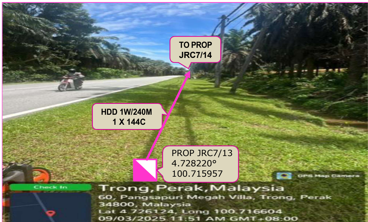
PROP 144C CABLE ROUTING VIA PROP JRC7/13 AT JALAN BESAR (ROADSIDE)
