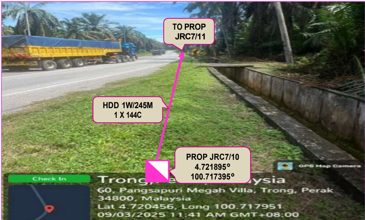
PROP 144C CABLE ROUTING VIA PROP JRC7/10 AT JALAN BESAR (ROADSIDE)
