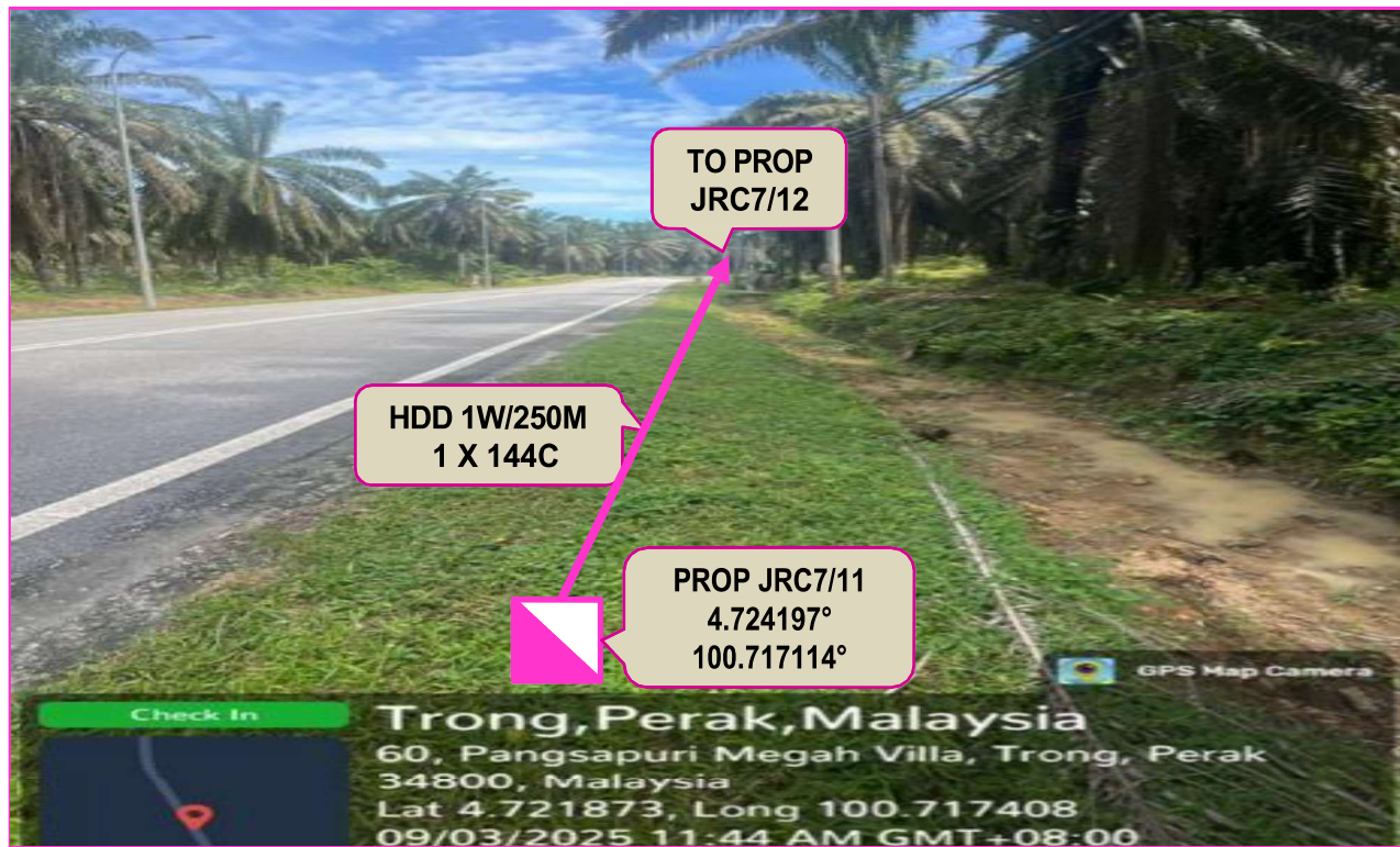
PROP 144C CABLE ROUTING VIA PROP JRC7/11 AT JALAN BESAR (ROADSIDE)
