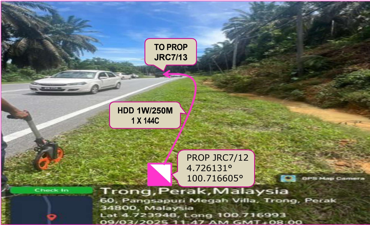
PROP 144C CABLE ROUTING VIA PROP JRC7/12 AT JALAN BESAR (ROADSIDE)
