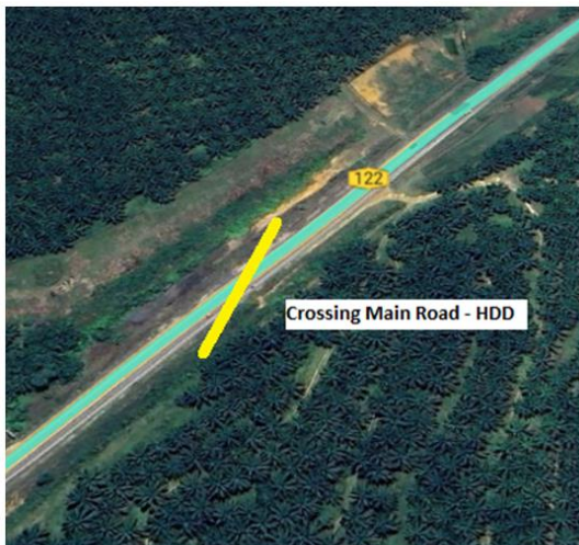
Crossing Main Road – HDD ( 4.585117° 103.335713°)
