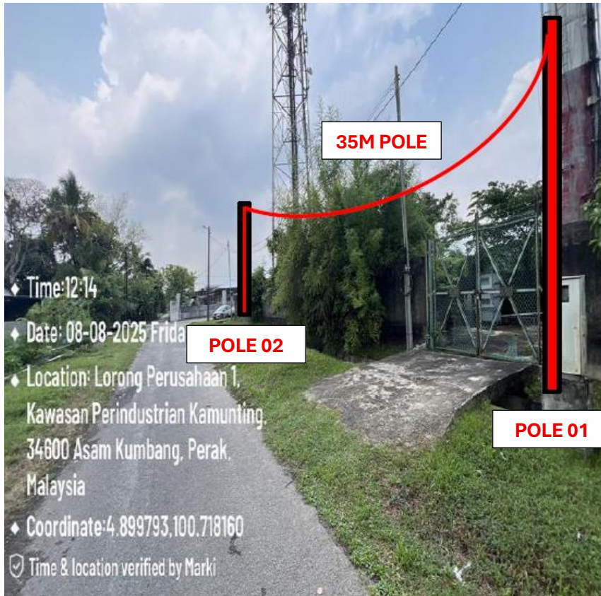
PICTURE 3 : POLE 01 TO POLE 02
