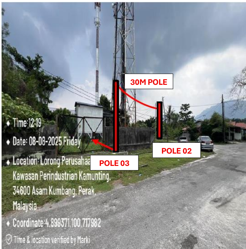
PICTURE 4 : POLE 02 TO POLE 03
