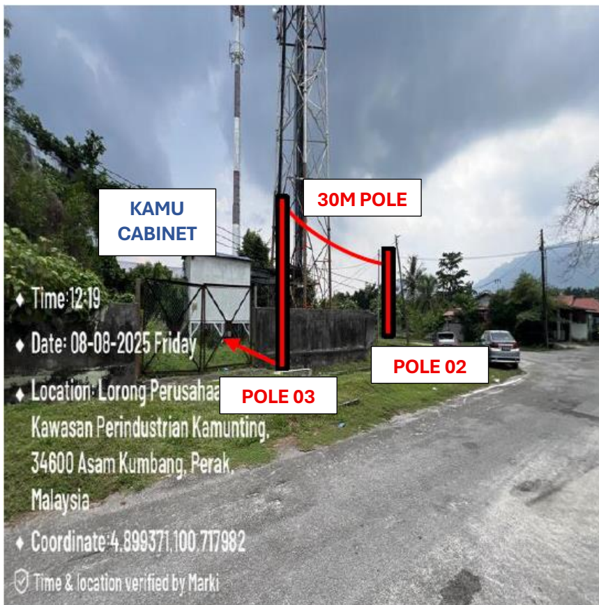
PICTURE 4 : POLE 02 TO POLE 03
